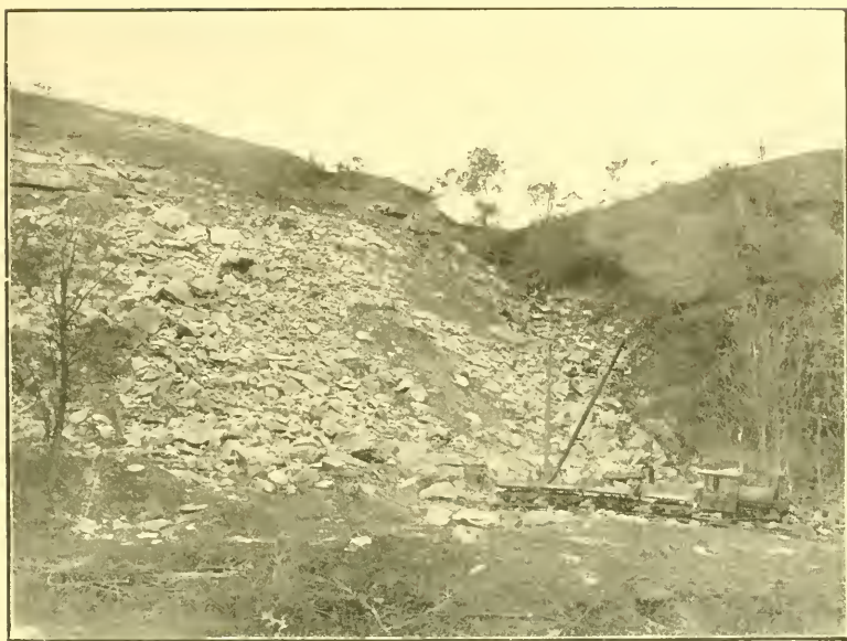
Old Falling Rocks, Bridgeport. Keller & Crossan, Contractors, tore all of these rocks down with one massive blast
